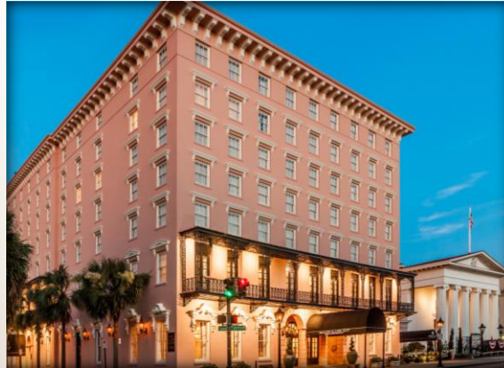
THE MILLS HOUSE HOTEL CHARLESTON
