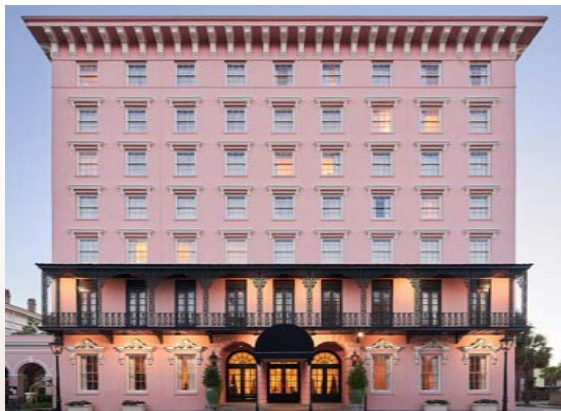
THE MILLS HOUSE HOTEL CHARLESTON
