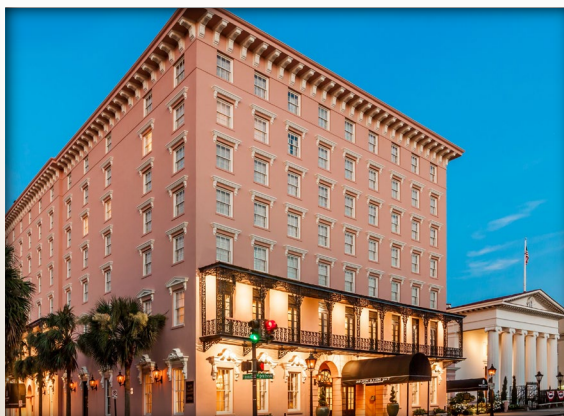
THE MILLS HOUSE HOTEL CHARLESTON
