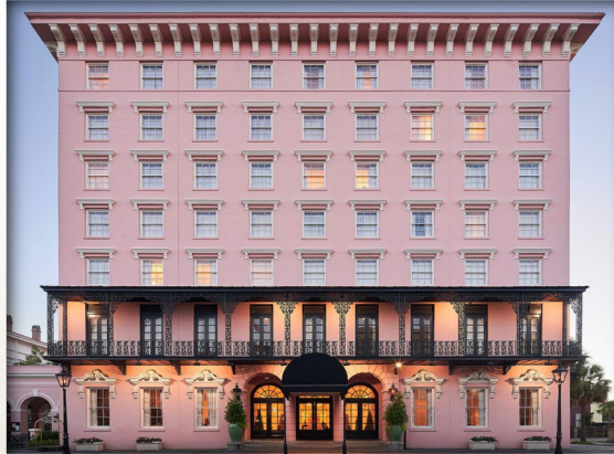
THE MILLS HOUSE HOTEL CHARLESTON
