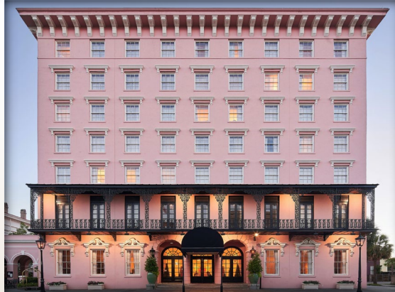
THE MILLS HOUSE HOTEL CHARLESTON
