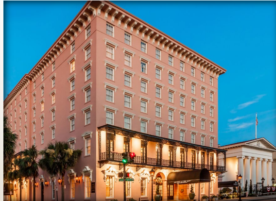
THE MILLS HOUSE HOTEL CHARLESTON
