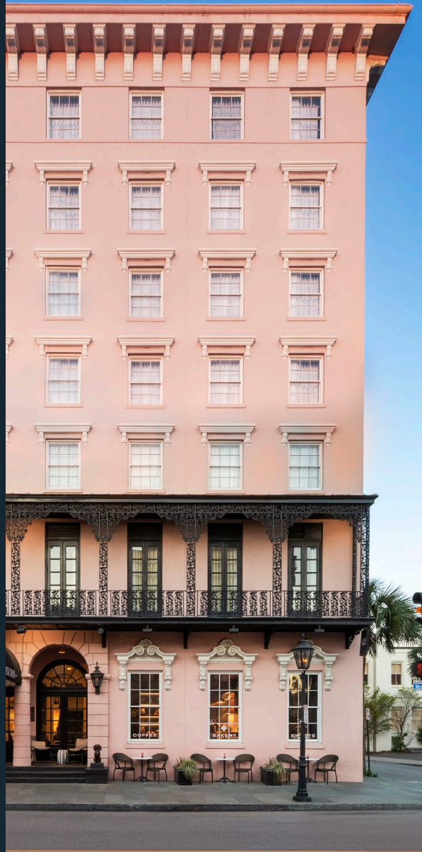
THE MILLS HOUSE HOTEL CHARLESTON
