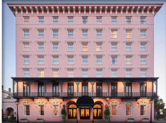
THE MILLS HOUSE HOTEL CHARLESTON
