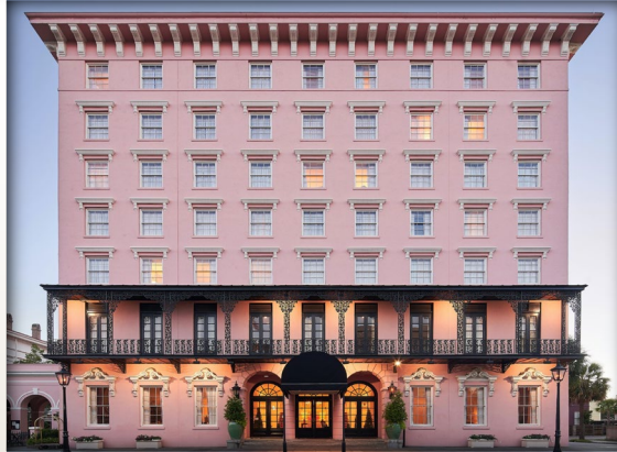
THE MILLS HOUSE HOTEL CHARLESTON
